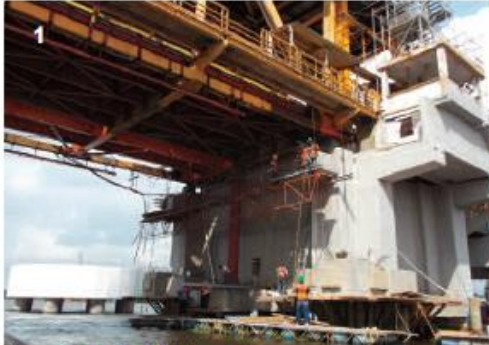
Above: Detail of the old bridge section
