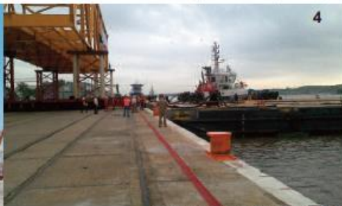
Above: Load out operation onto 2 barges
