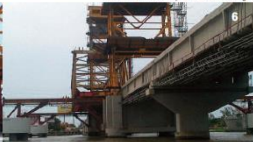
Above: Detail of the old bridge section skidded on one side
