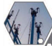
8 X L180 JACKS MOUNTED ON STOOL ON CRANE LEGS
