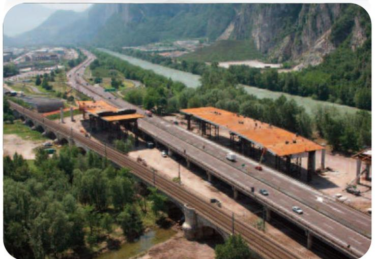
The two sections were secured by the Spmt's and safely loaded. The extensive work before installation involved physical movement and stability studies, and risk assessments of possibilities as unlikely as a vehicle accidentally running off the road and on to the worksite.
