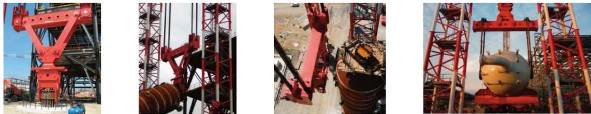
**TAILING WITH SPMTs - CRAWLER CRANES - SKID SHOES AND TAILING FRAME**
