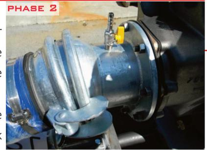
**PHASE 2:** To make easy the hose removal, open the air inlet valve in order to restore the atmospheric pressure inside the hose and discharge the water column. Before the removal of the hose, close the air inlet valve.
