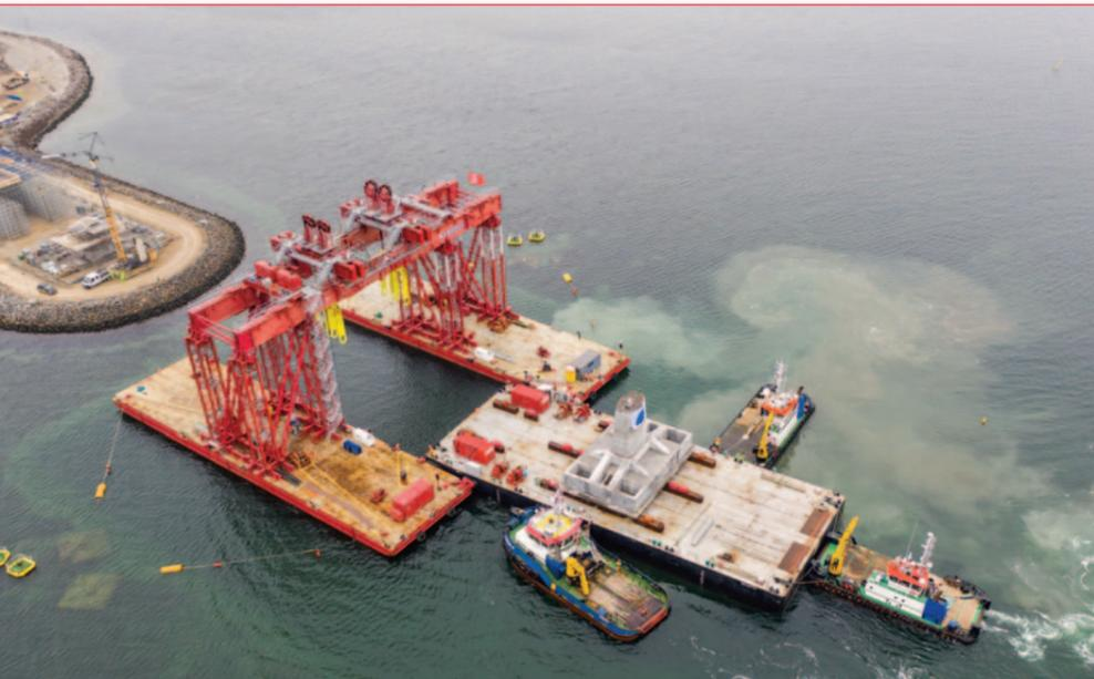
Fagioli Catamaran has several applications in the offshore sector thanks to its revolutionary construction based on barges and tower systems provided with crosshead beams and strand jacking system. By means of the skid shoes it is possible, keeping the catamaran in the same position, to move the load (the prefabricated foundation) in the plane, in both directions, in such a way to achieve a very accurate positioning of the foundation,
