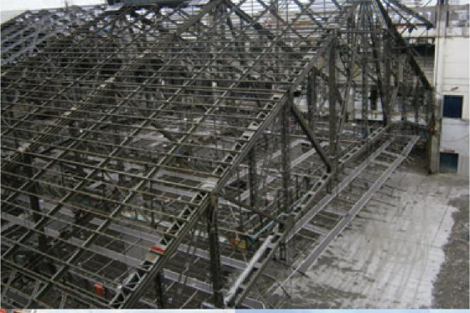
The 25m lowering was performed by fourteen Fagioli L180 lifting / lowering jacks, mounted on cantilever beams (temporary structure) which in turn were on top of the permanent columns; each strand jack was assisted by an individual PPU. Four Fagioli L50 guy jacks in frames were mounted on each corner of the building to control any possible horizontal deviation of the roof during the operation.
