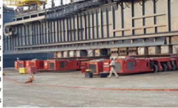
the load was transported towards the jack-up area near to jack-up skid beam. jack-up skid beam height and onto skid beam clamps (by the SPMTs) the item system at 2 m distance. The required to Fagioli scope of removing lines as the position (pictures at the top
