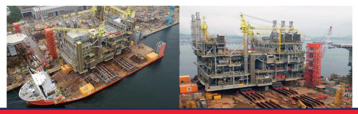
Top: Load out operation of a 44,000 ton section in Korea by means of 64 skid shoes (1000 t capacity each) Bottom: Load in and transport, lifting skidding and final installation of modules for the intersection operation
