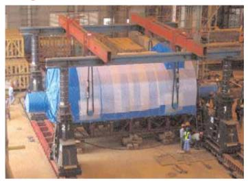
Construction of Cilegon CCPP in Indonesia involved the installation of a Starting Unit, Generator and Gas Turbine using a Fagioli PSC Telescopic Gantry.
