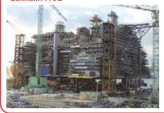
Further to our last Newsletter we have now transferred the loads for both the LUN/A and PA/B topsides for Samsung Heavy Industries so that they are now on four support points. Additionally, the weighing of both decks has now been completed with the LUN/A deck weighing 15,900 tonnes and the PA/B deck weighing 22,100 tonnes. The main lifting operations are scheduled to commence in March 2006 starting with the LUN/A deck which may have gained a little weight to 23,500 tonnes.
