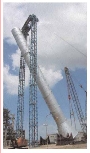
The Fagioli Group performed the transportation and erection of a C-3 Splitter, weighing 1,500 tonnes, 98 metres long and 14 metres diameter for Reliance Industries Ltd. The splitter was manufactured by Doosan at their factory in Masan, Korea and shipped across the Indian Ocean.
