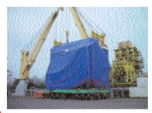
The first stage was the transportation of the boiler 13.72 metres x 8 metres x 11.54 metres weighing 230 tons from Taranto NE / CCT premises to Taranto port using 2 x10 axles SPMTs. Other parts were assembled onto the structure with a different configuration reaching a width of 11.15 metres and a weight of 350 tons.
