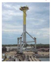
In Ravenna, Italy Fagioli performed a couple of interesting loadouts: a 900 tonne Jacket tripod (left picture) by means of 3 x 12 axles SPMTs and a 425 tonne deck (right picture) moved by means of 2 x 12 axles SPMTs.
