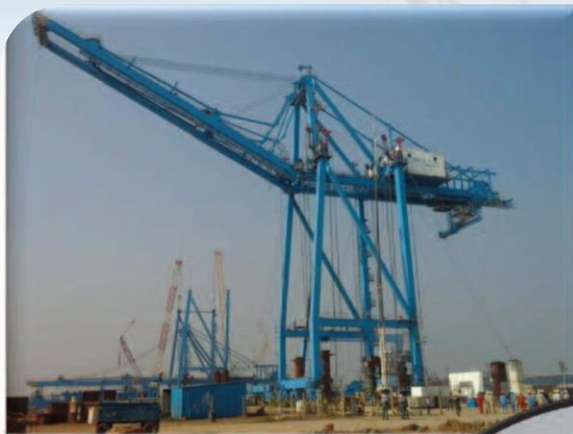
Final Lifting Position
