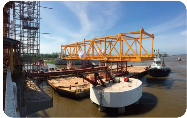
Above: detail of bridge load out onto 2 barges
