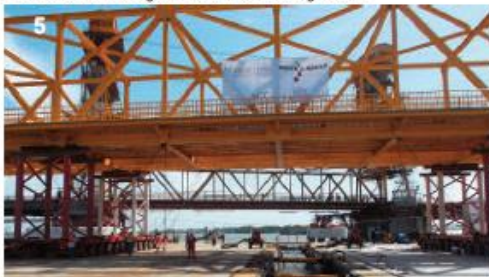
Above: Arrival of the barges and bridge section at installation area
