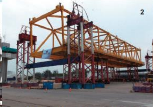
Above: Detail of the new bridge section lifted by strand jacks
