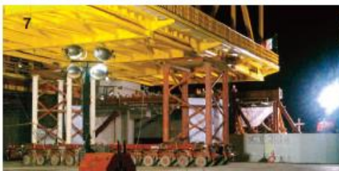
Above: Installation of the new bridge section
