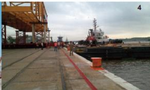
Above: Load out operation onto 2 barges
