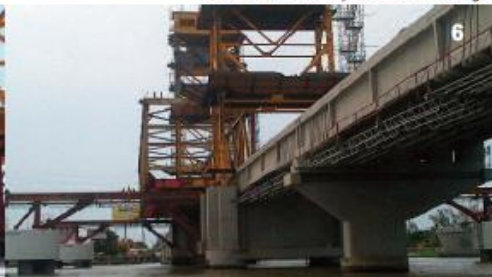
Above: Detail of the old bridge section skidded on one side
