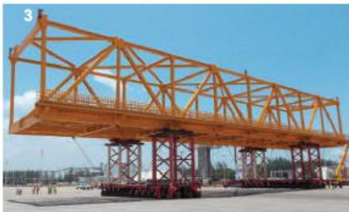
Above: SPMTs taking all the load of the bridge section
