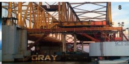
Above: The old bridge section is taking away
